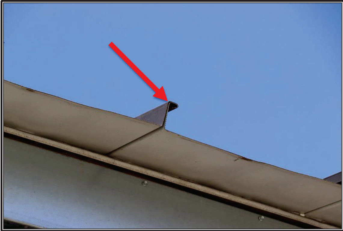
Photo 16: Representative view of a 90-degree single roll (1 phase) standing seam metal roof panel (arrow).
