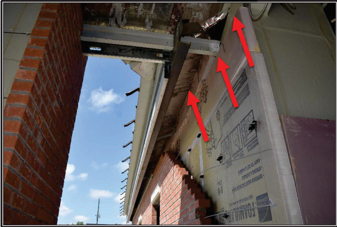
Photo 22: Representative view of missing spray foam insulation at the roof-to-exterior-wall interface (arrows).
