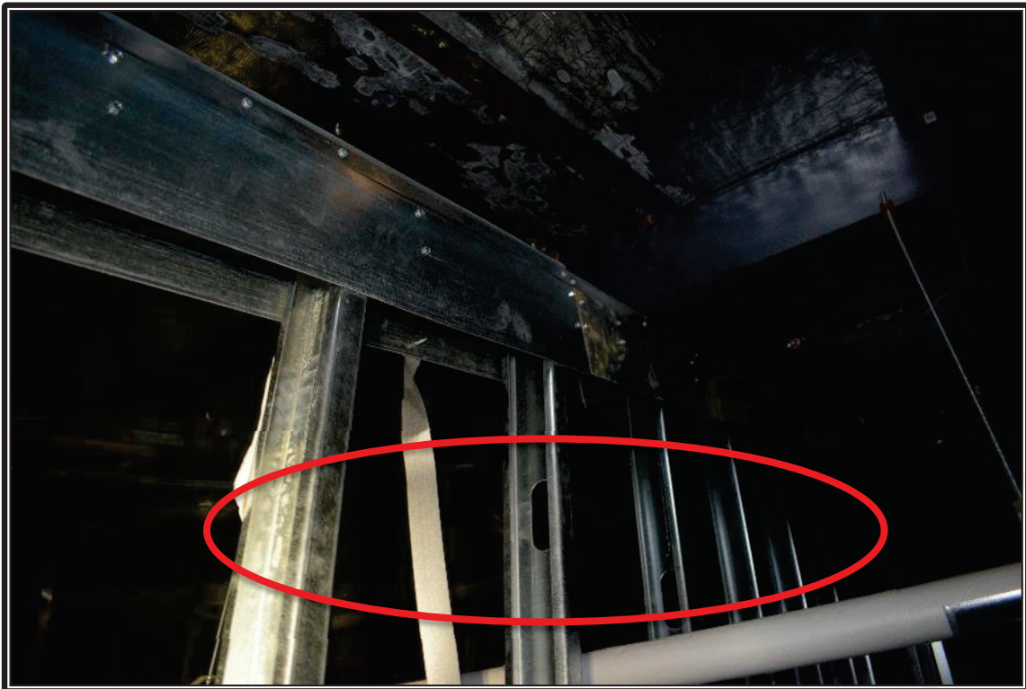
Photo 12: Representative view of the missing light-gauge metal wall bridging (oval).
