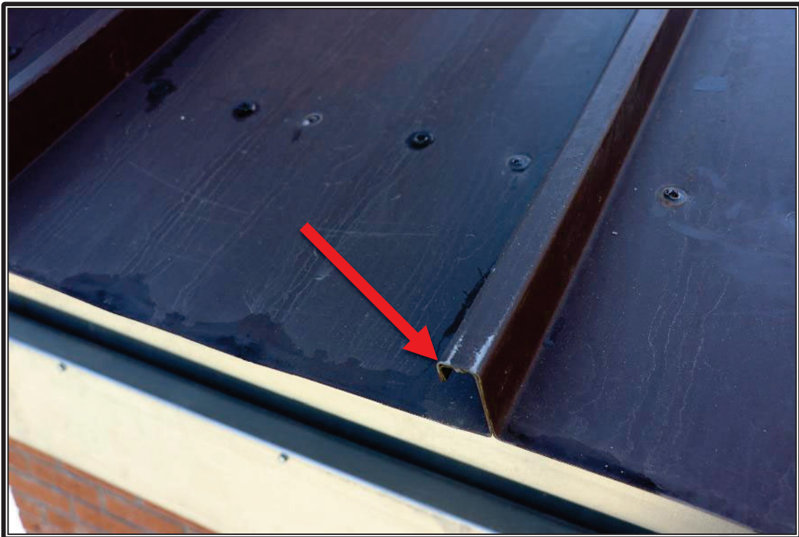
Photo 17: Representative view of an unseamed standing seam metal roof panel (arrow).
