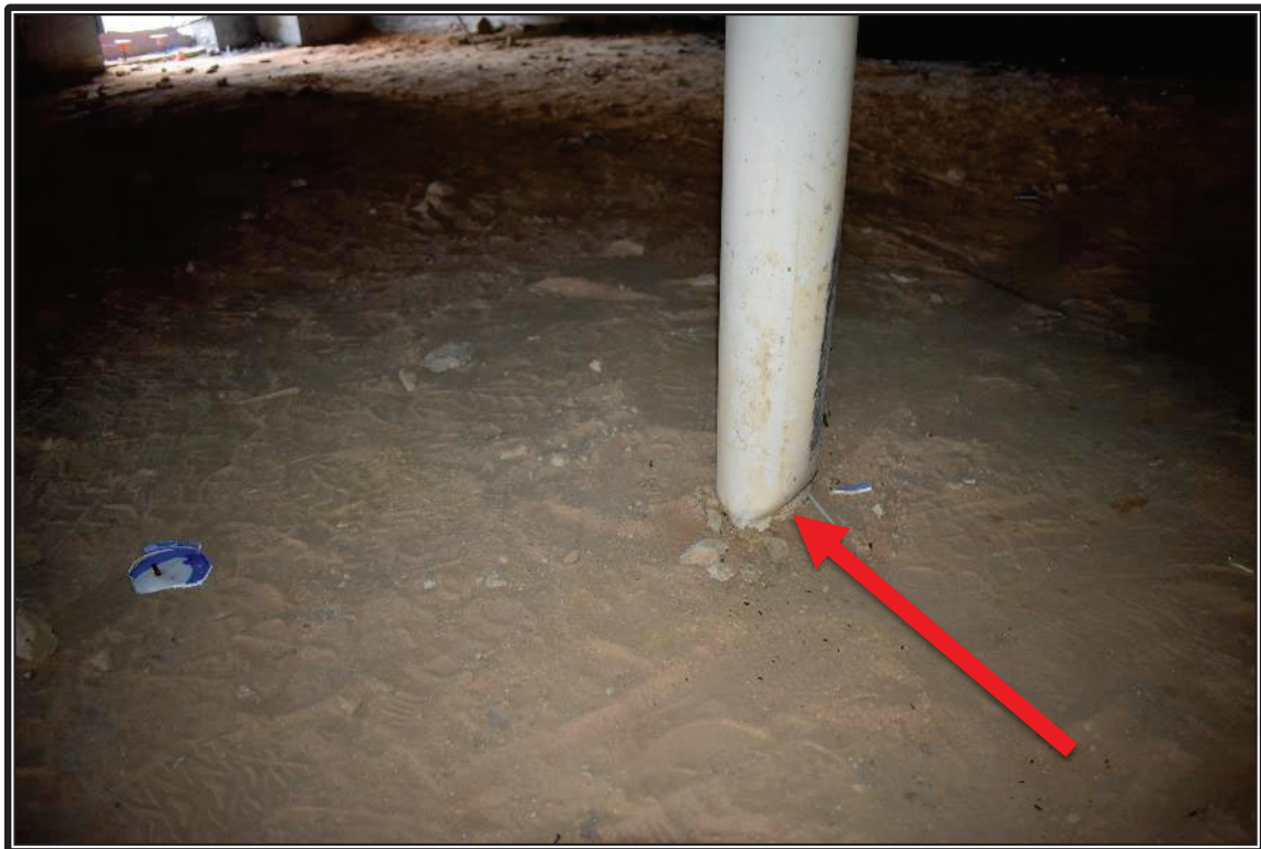
Photo 33: Representative view of partially bent over and collapsed pipe stub (arrow).
