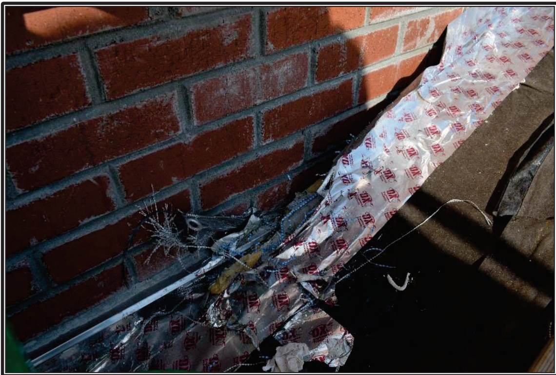
Photo 21: Representative view of through-wall flashing penetrating the roof insulation.
