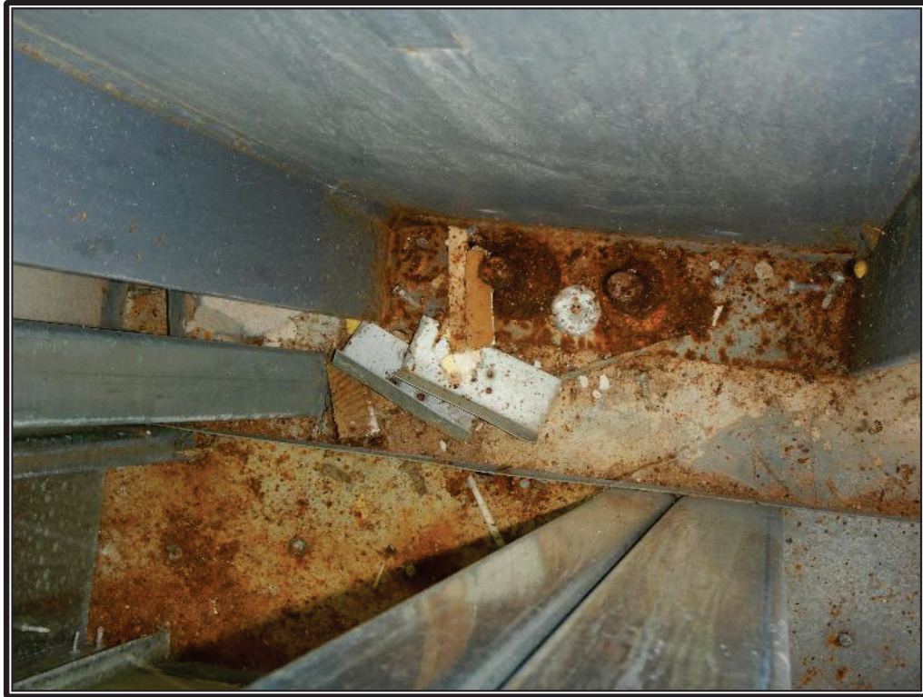
Photo 26: Representative view of the bolts and structural steel with surface corrosion.
