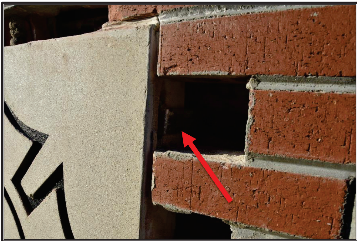
Photo 8: Representative view of the anchor at Test Area 2 (arrow).
