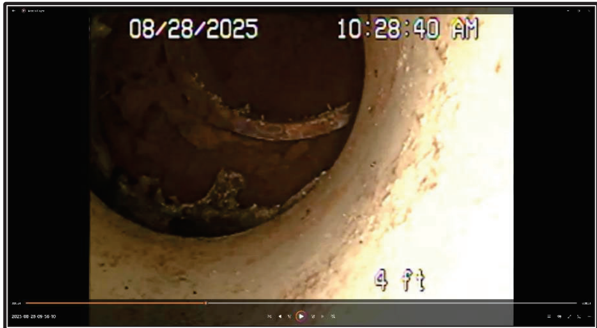
Photo 32: Representative view of a separated/cracked/collapsed section of pipe (courtesy of Next Level).
