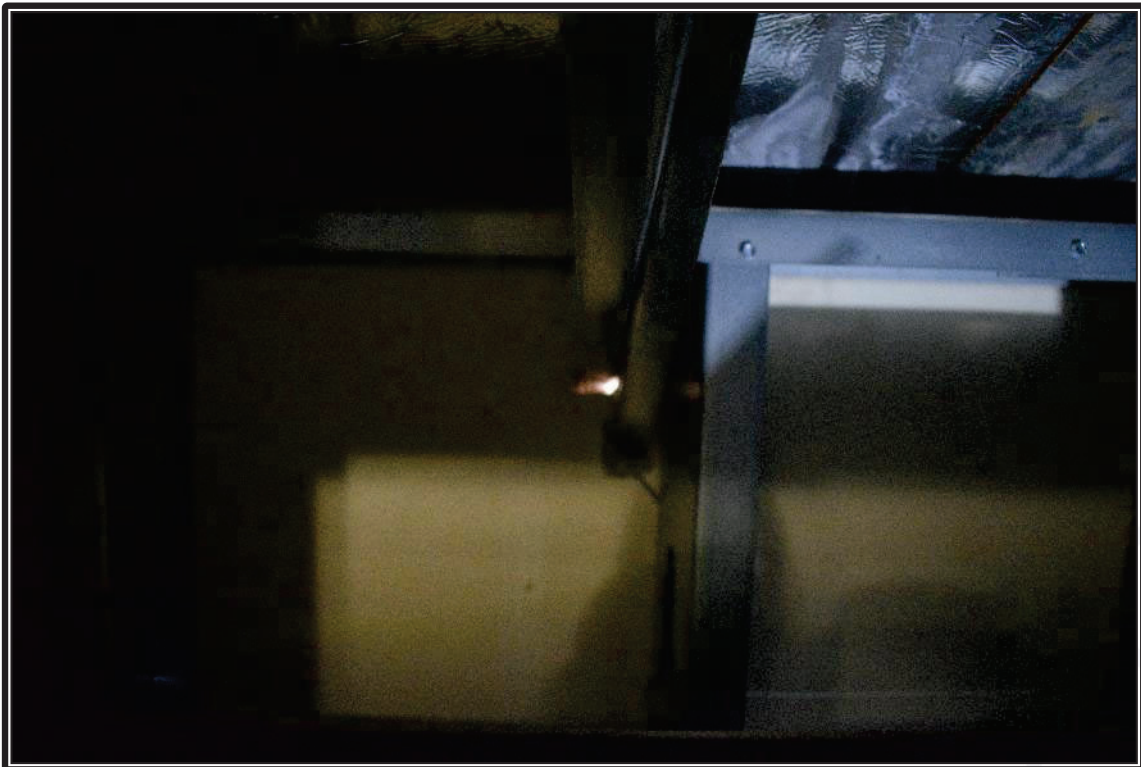
Photo 23: Representative view of visible daylight through an unsealed penetration at the exterior wall sheathing.
