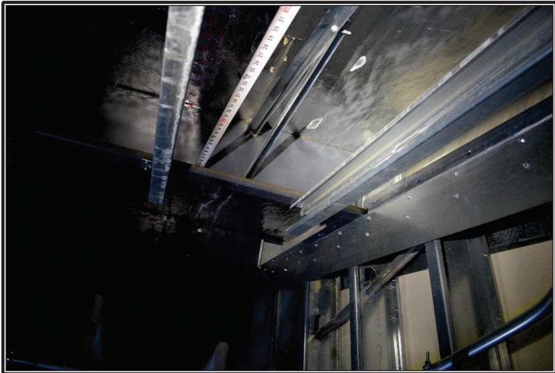
Photo 10: Representative view of the metal strapping at the slip track.
