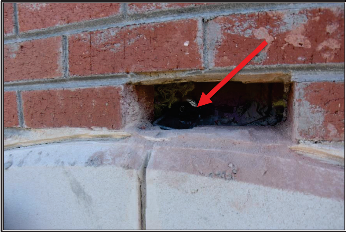
Photo 9: Representative view of a masonry wall tie at the head of the window opening at Test Area 3 (arrow).
