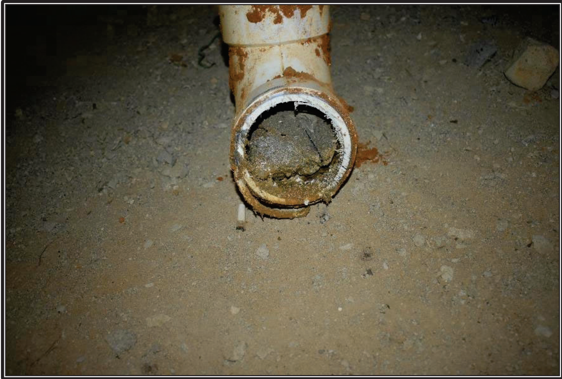
Photo 30: View of debris/dirt/stone-filled pipe.
