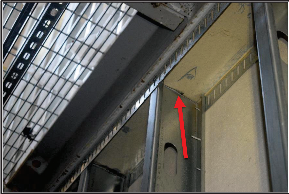
Photo 11: Representative view of a light-gauge metal stud with inadequate clearance at the slip track (arrow).
