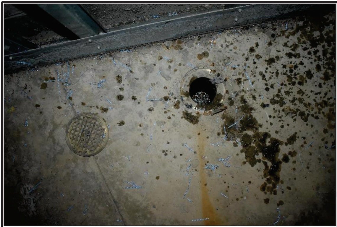
Photo 29: Representative view of a pipe filled with a watery sludge.
