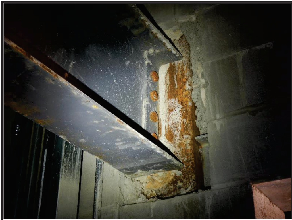
Photo 27: Representative view of the bolts and structural steel with surface corrosion.
