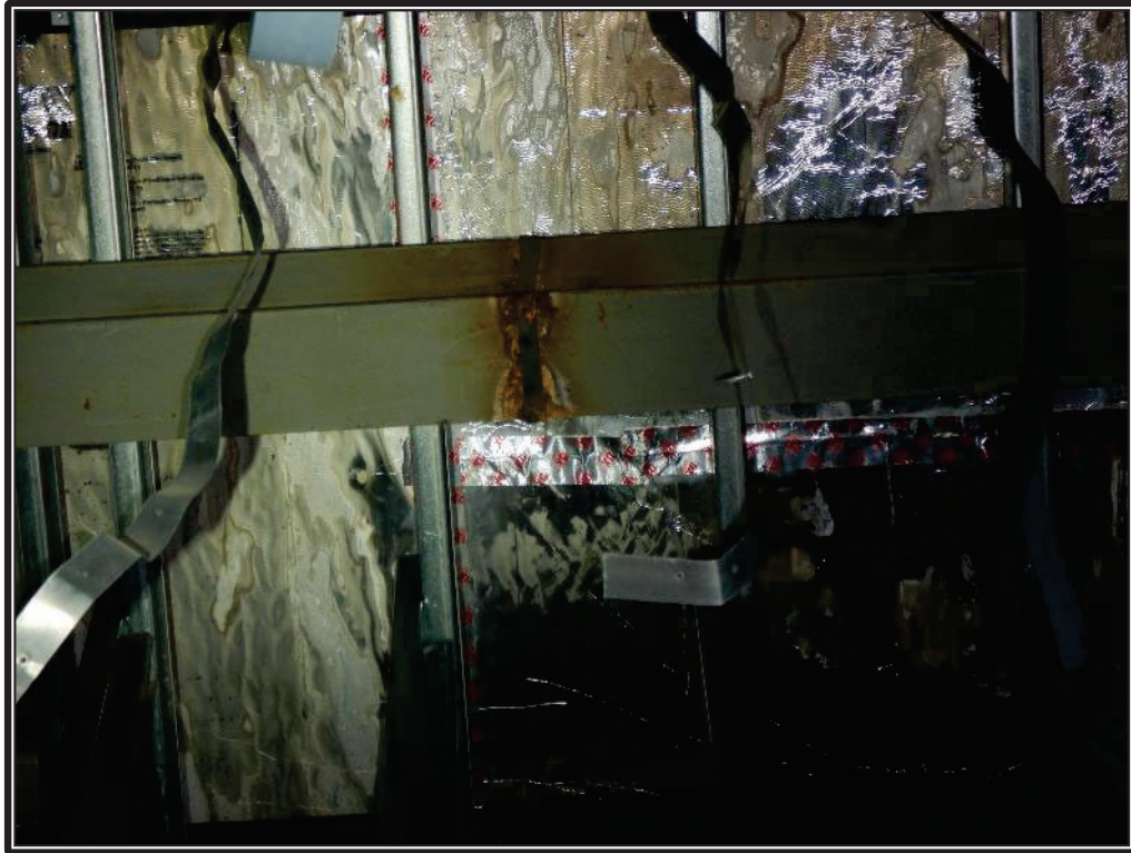
Photo 24: Representative view of an apparent uncoated field weld with surface deterioration at a PEMB beam splice.
