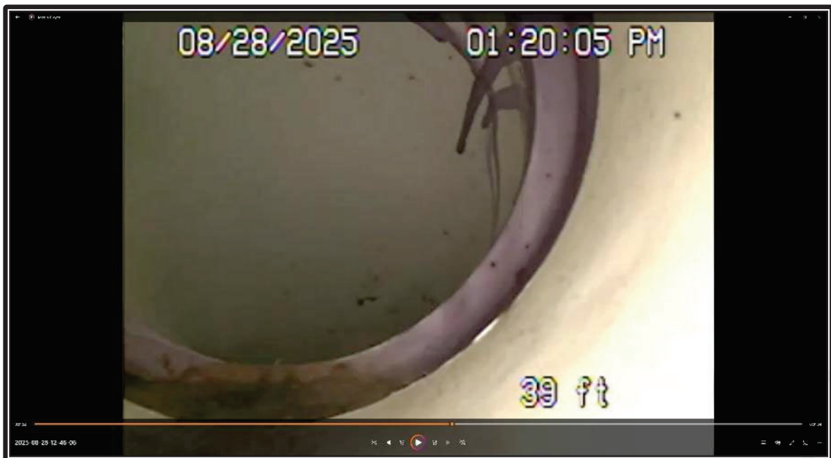
Photo 31: Representative view of a partially separated or poorly fit pipe joint (courtesy of Next Level).
